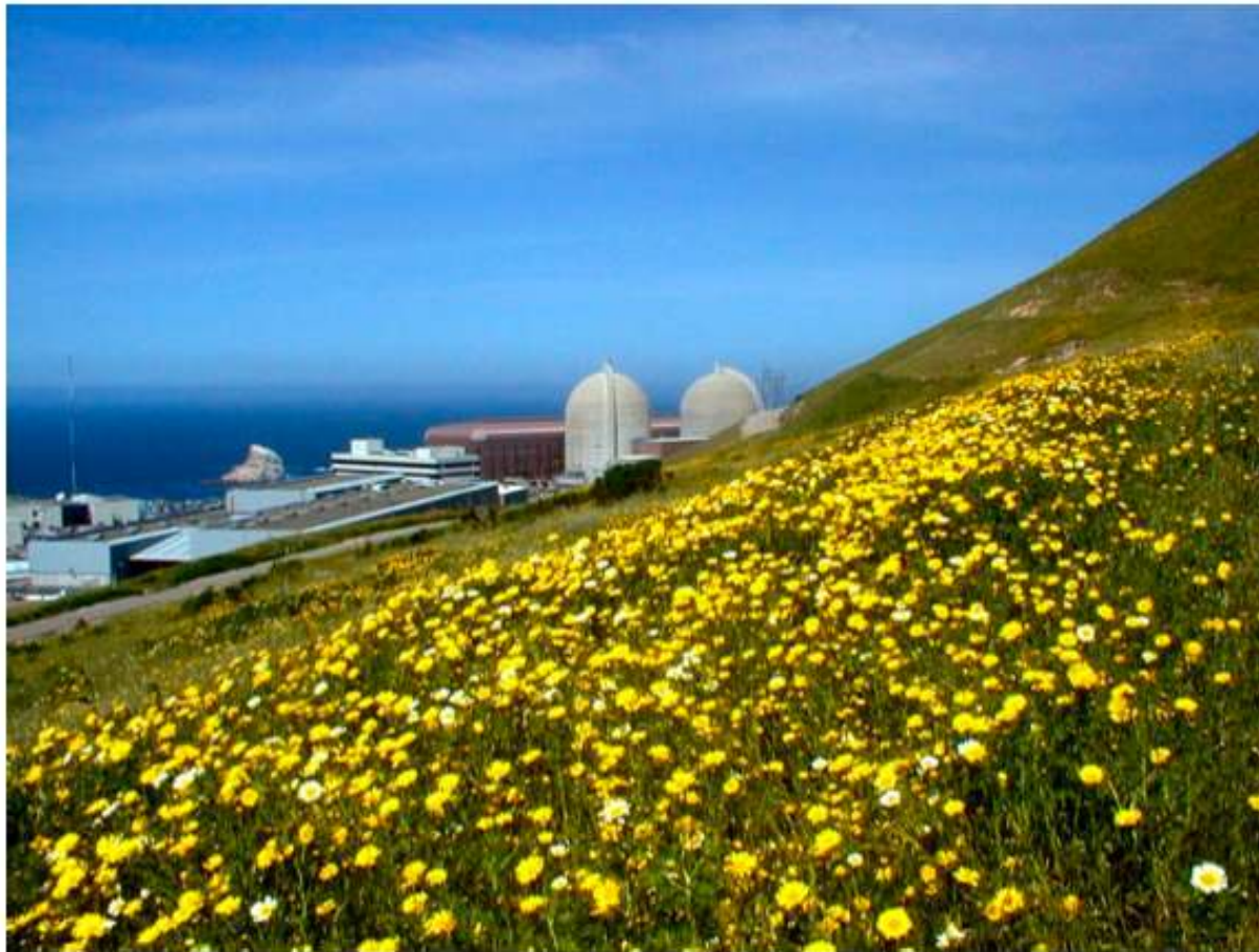
Spring wildflowers at the Diablo Canyon nuclear power plant
